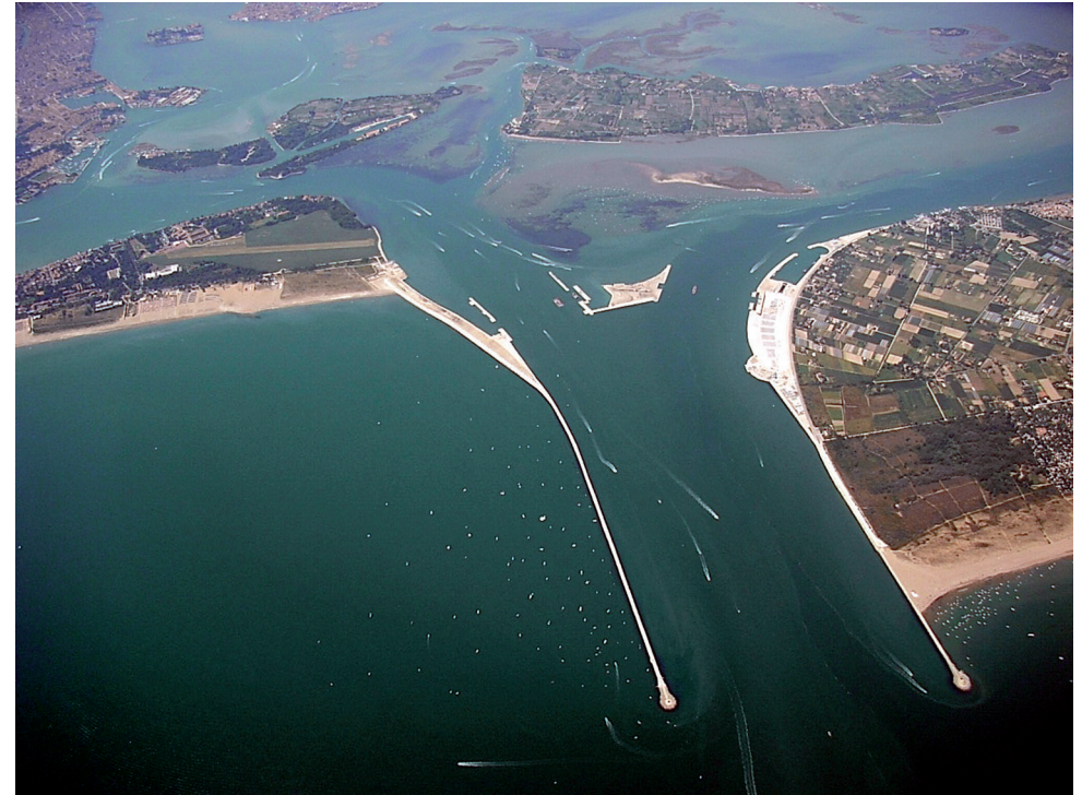
© Chris 73 - Aerial view of the Lido lagoon inlet with construction of the MOSE mobile barriers
